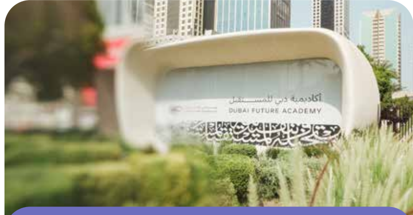
3D Printed Office Classroom
